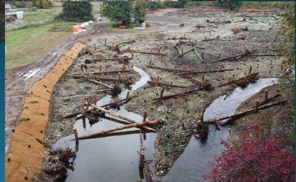
Upper Royal Arch Floodplain and Habitat Restoration Project – Cedar River
