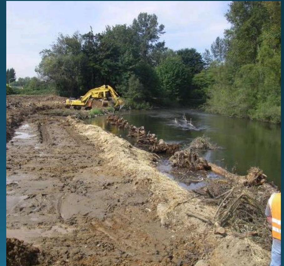
Fenster Levee Setback, Auburn
