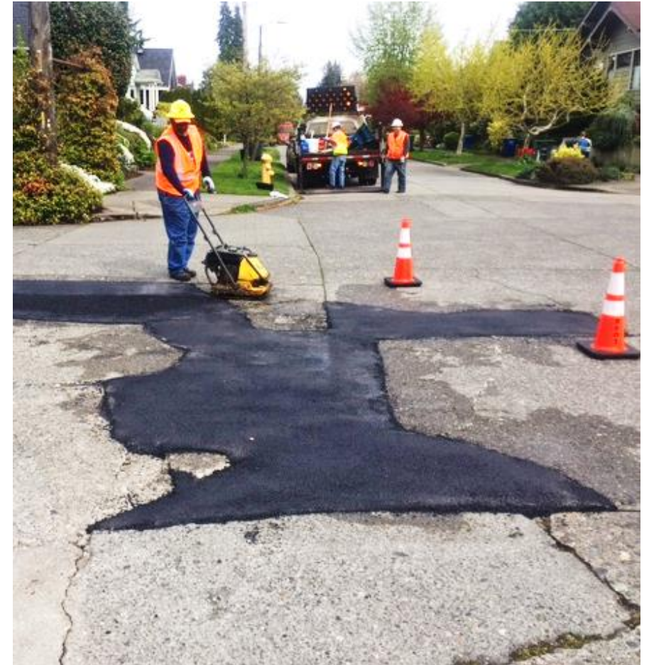
Crews repairing potholes
