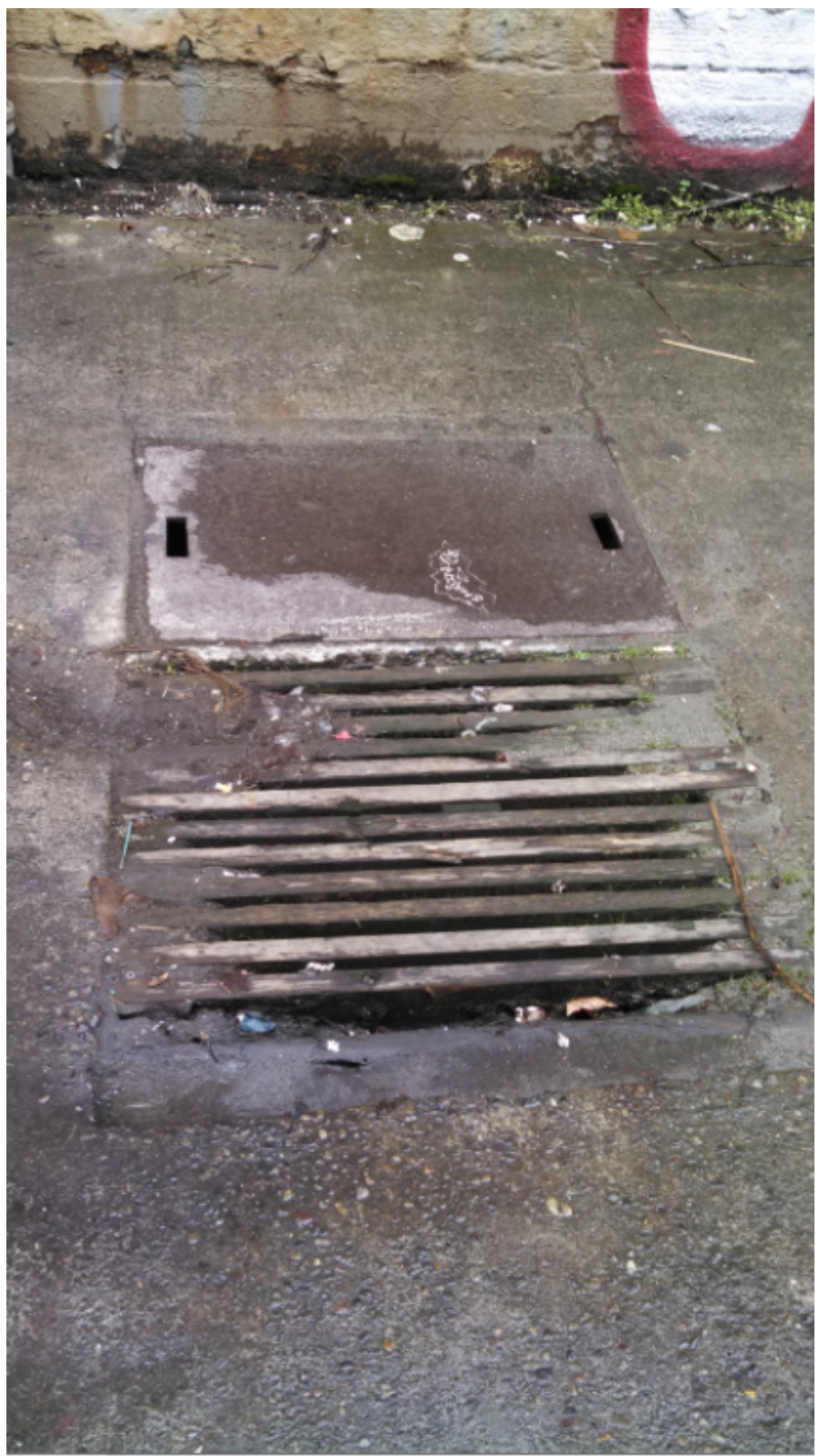
Drainage structure with wood grate
