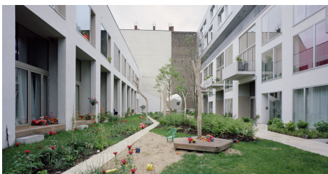
A courtyard incorporates area for trees and play space for kids, with direct sightlines to units.
