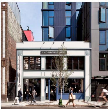
New development incorporates a historic facade and mid-block passageway. The two-story facade provides a transition from the taller building to a pedestrian scale and breaks up the building massing.
