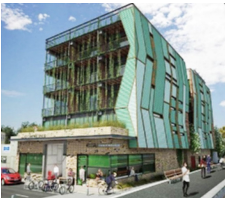
An appropriately-scaled brick base provides grounding for a set-back upper massing. Balconies provide depth to the facade while a skilled use of analogous colors adds a whimsical flair that is not overwhelming.
