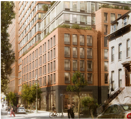
Base massing reflects the immediate context with the use of brick and fenestration patterns. Setbacks and modulation reinforced with changes in the design language.
