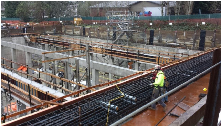
Windermere CSO storage tank
