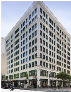
Joshua Green Building, 1425 4th Ave Seattle
