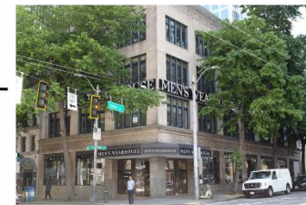
Great Northern Building 1404 4th Ave, Seattle
