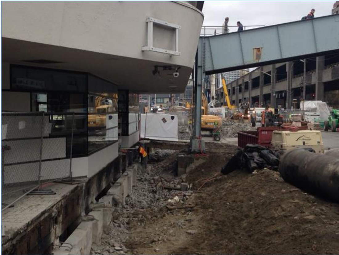
(Seawall demo, looking north from the Ferry Terminal entrance)
