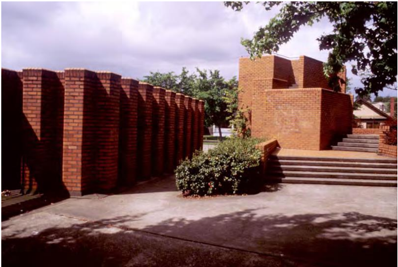
East Pine Substation, 1501 23 rd Avenue, 1969
