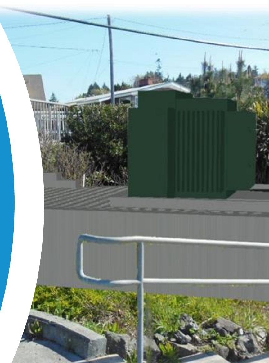
King County Alki Transformer
