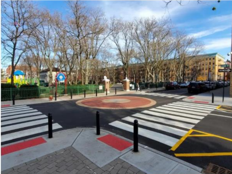
A raised intersection at Ninth and Grand streets along with new crosswalk with wide stripes and reflective paint. Photo: City of Hoboken
