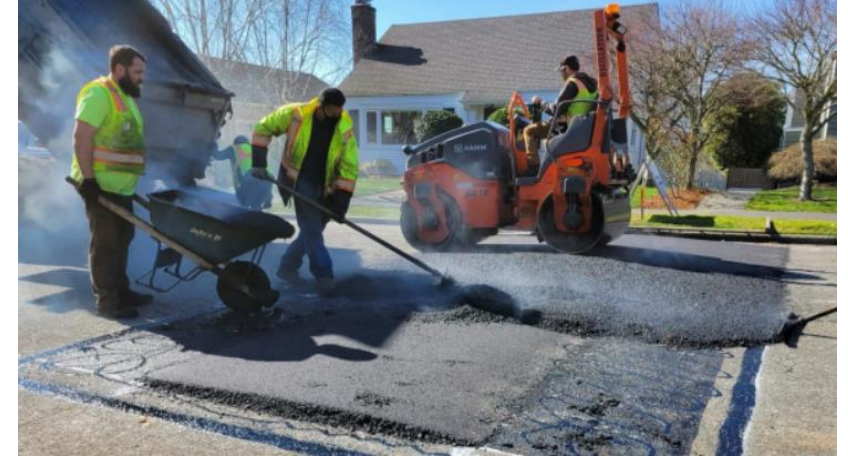
SDOT team installing speed cushions along the W Seattle Neighborhood Greenway
