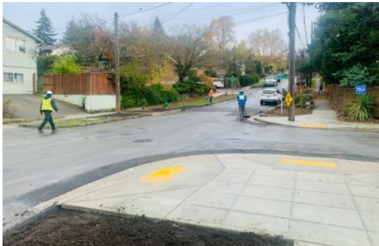
New curb ramps, upgraded sidewalks near Wing Luke Elementary
