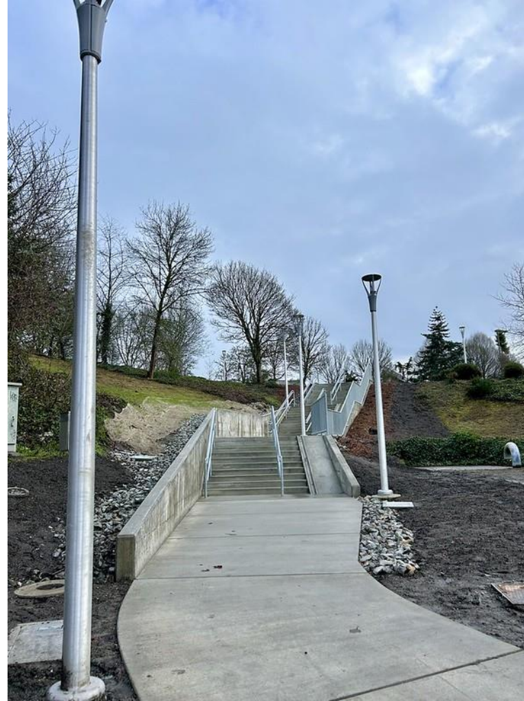
I-90 – Judkins Lighting and Staircase
