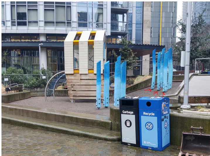
Urban Triangle Park Play Area - under construction
