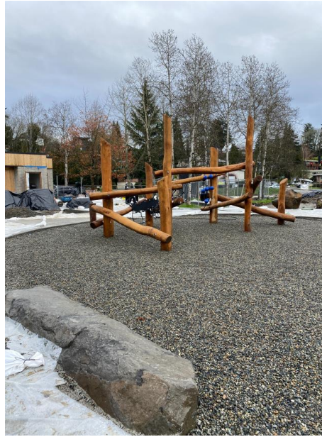
Pathways Park – under construction
