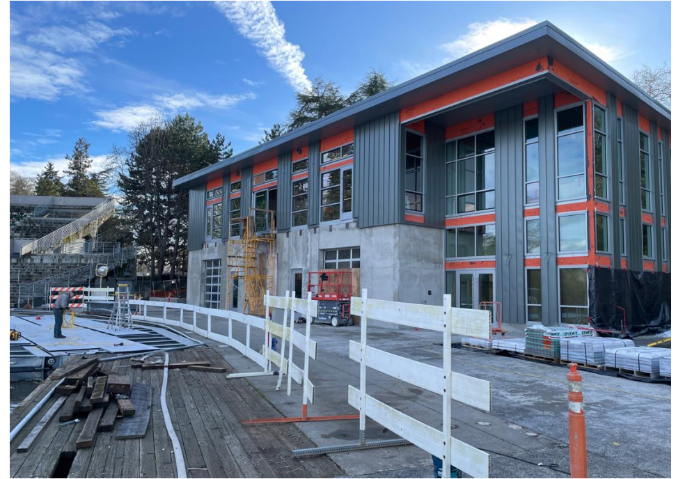
Green Lake Small Craft Center – under construction
