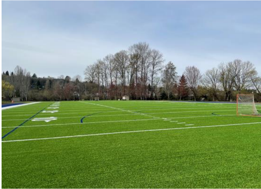
Montlake Community Center Playfield - completed
