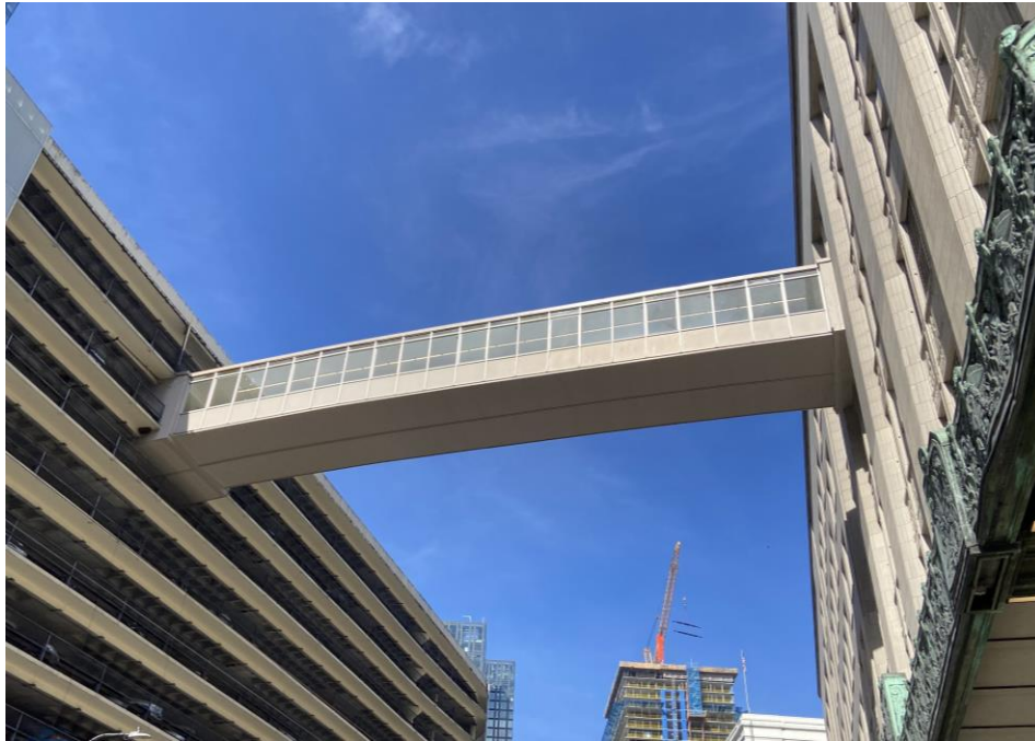
Exterior looking south
