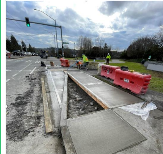
Construction crews paving new southbound bike ramp at I-90 Trail. Photo SDOT.
