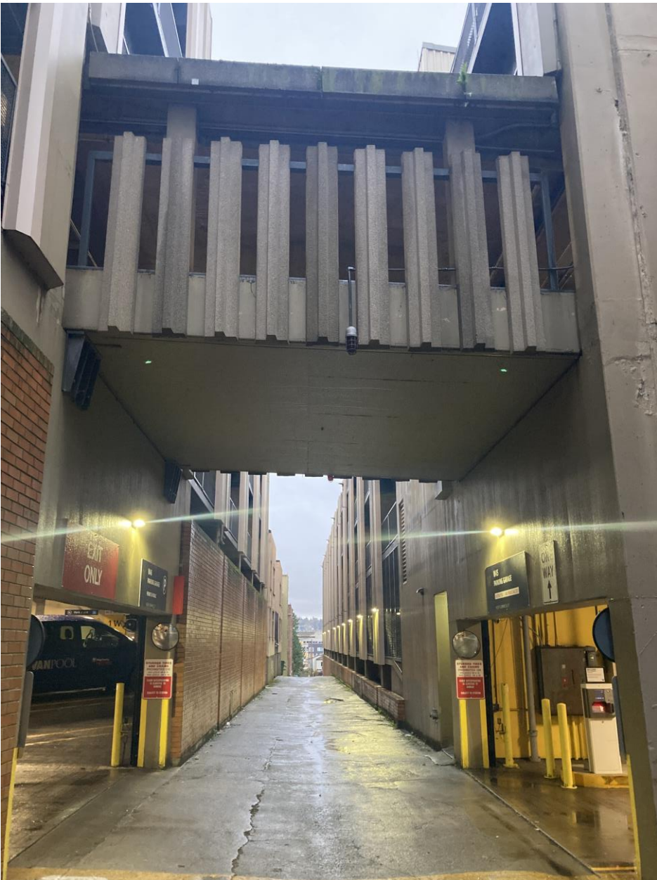
Summary Att B - UW 12th Ave NE Alley Skybridge Photos V1
