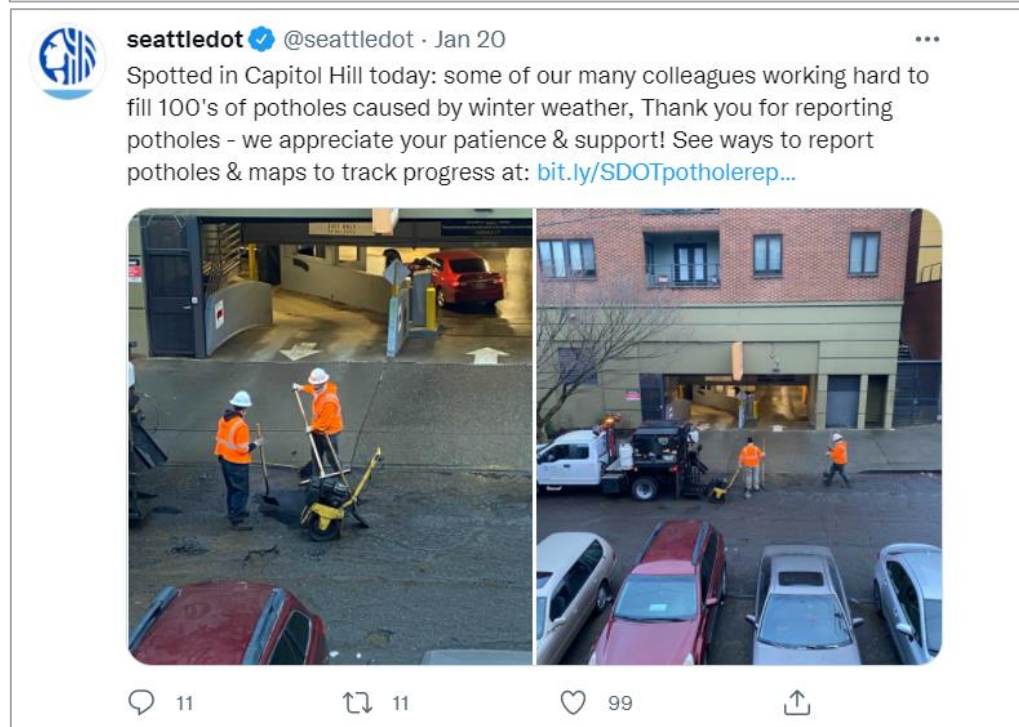
SDOT Tweet: Pothole repair work in Capitol Hill
