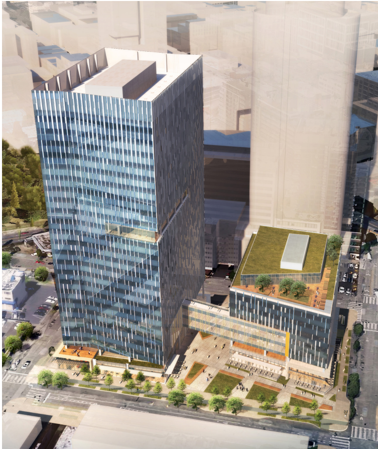
View Looking North
