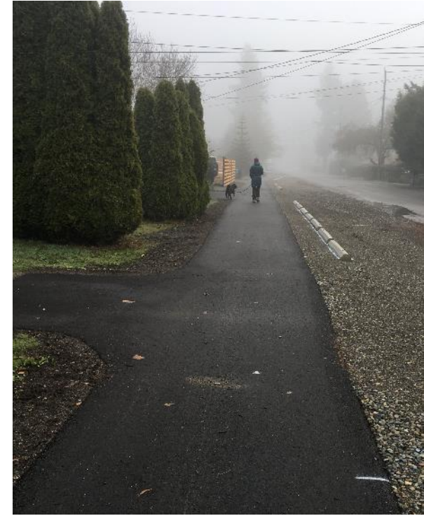
Cost effective walkway: NE 135 th St between 15 th Pl NE and 20 th Ave NE
