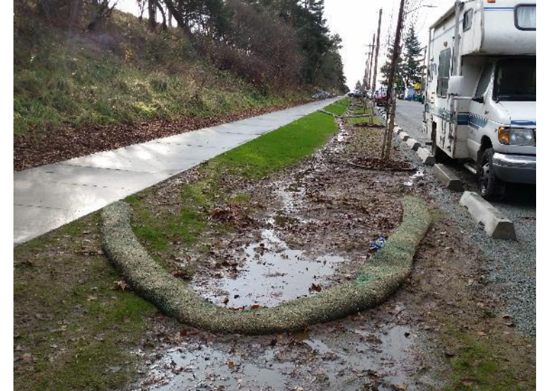
At-grade concrete: 16 th Ave S – S Dakota St to S Nevada St
