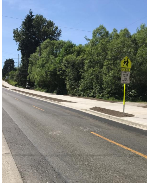
New sidewalk: S Orcas St between 26 th Ave S and 32 nd Ave S
