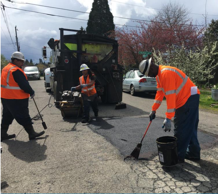
Maintenance paving, such as panel replacements and filling potholes
