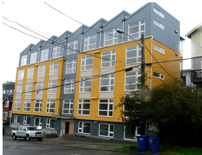
Front of building.
