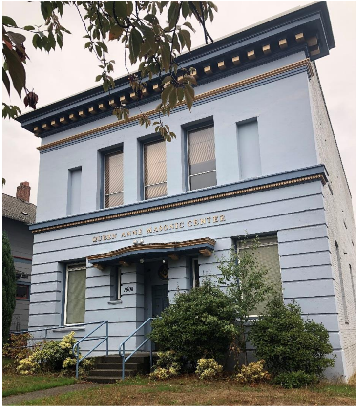
Sunset Telephone & Telegraph Exchange, 1608 4 th Avenue West, 2018
