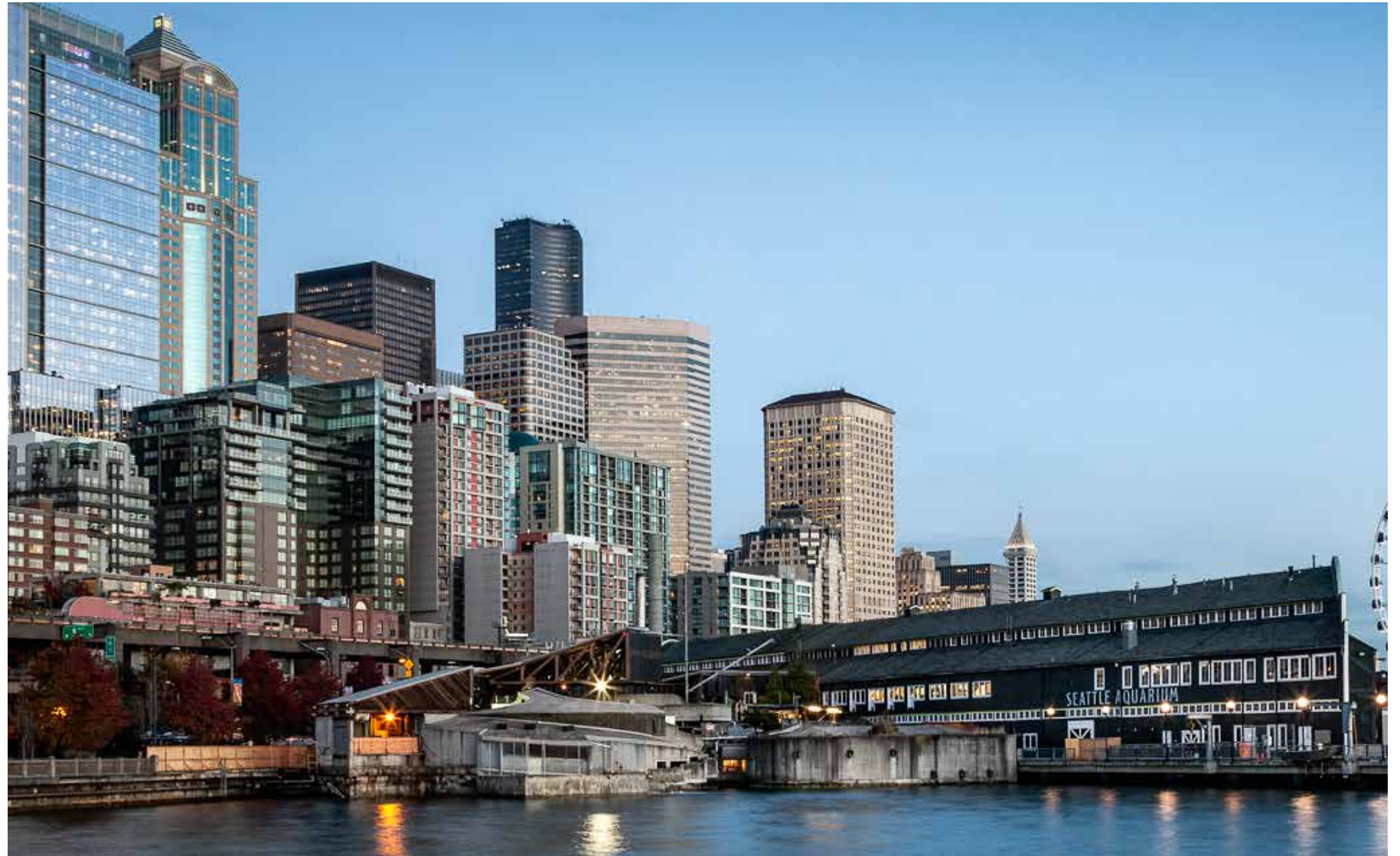
View of the Seattle Aquarium after finger pier was removed for replacement in 2014.
