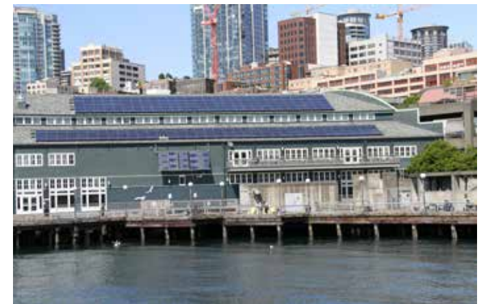
247-solar panel installed on the roof of Pier 59 in 2013.
