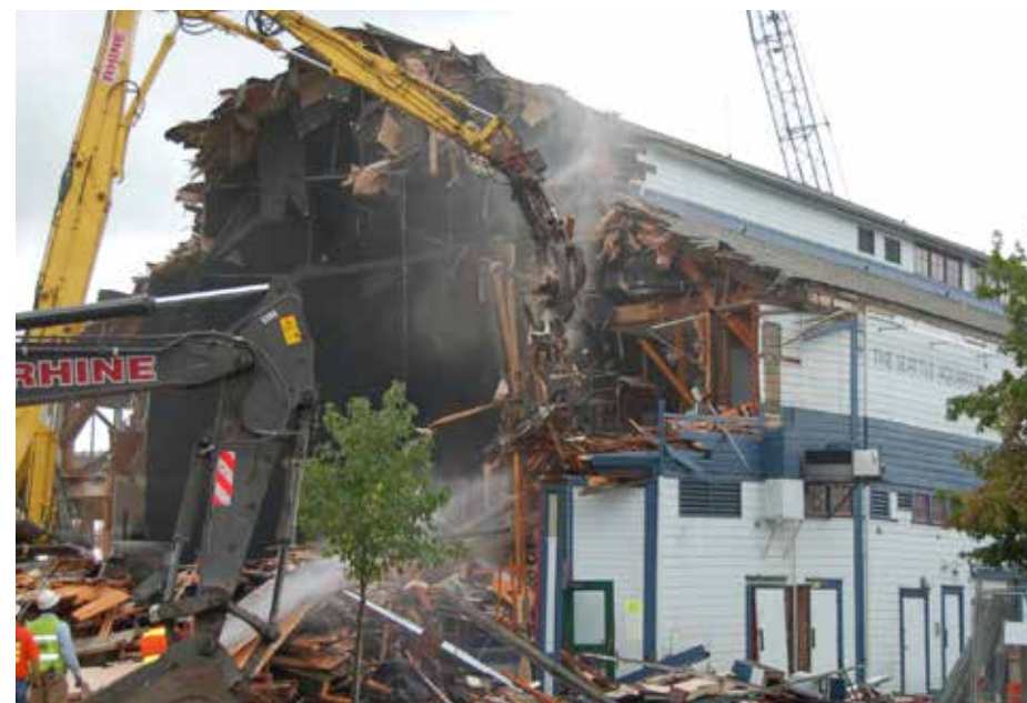
Demolition of the west end of Pier 59.
