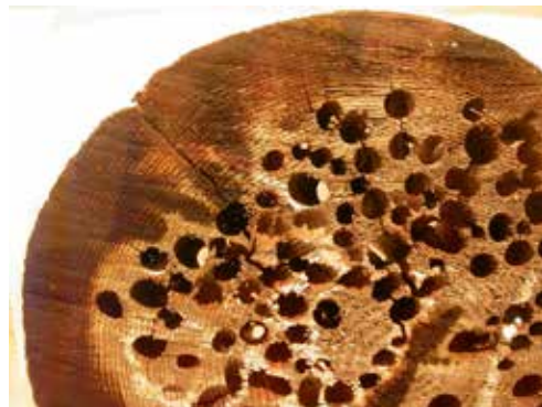
In 2007, Pier 59 renovation replaced over one thousand compromised wood pilings.
