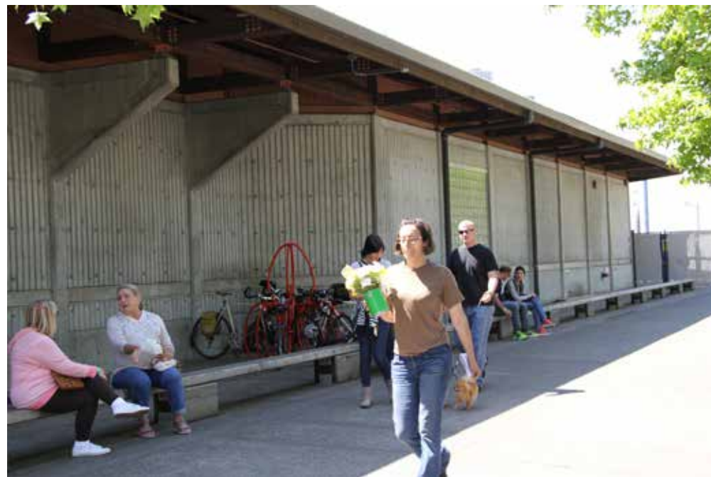
Renovation of Pier 60 could increase views in and out of the building.
