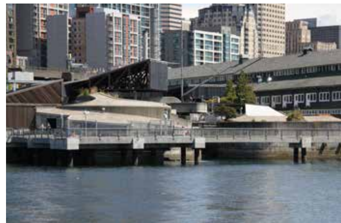
Pier 60 after new harbor seal exhibit and finger pier replacement in 2014.
