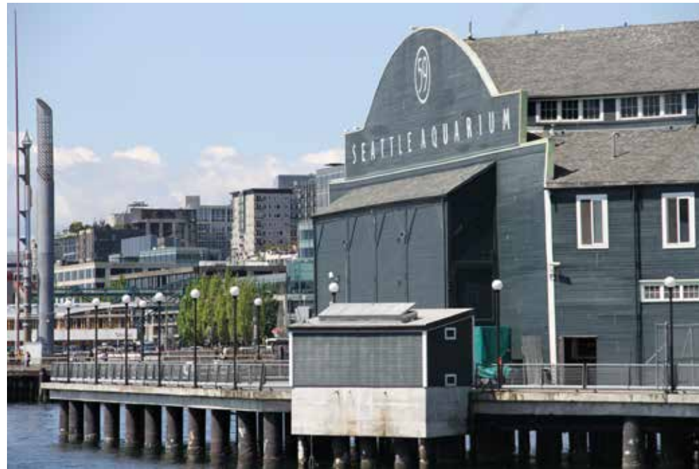
With renovation of Pier 59, the west facade could be opened up to maximize views.
