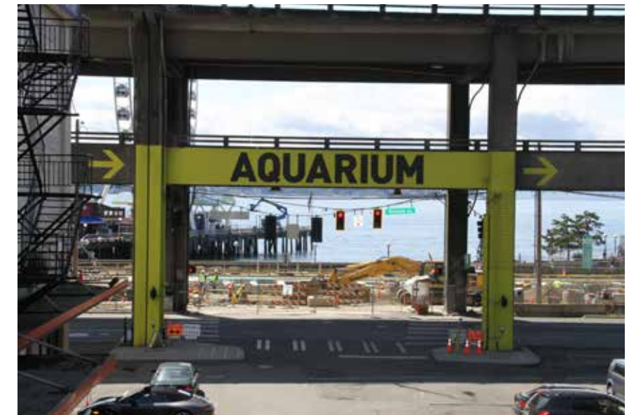
The existing Alaskan Way Viaduct separates downtown Seattle from its public waterfront.
