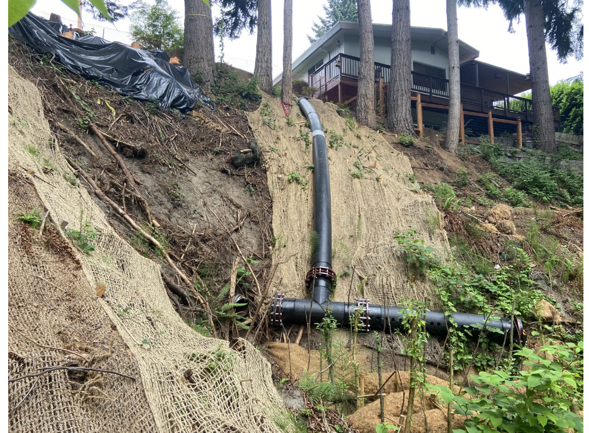
2023 – Temporary culvert installed
