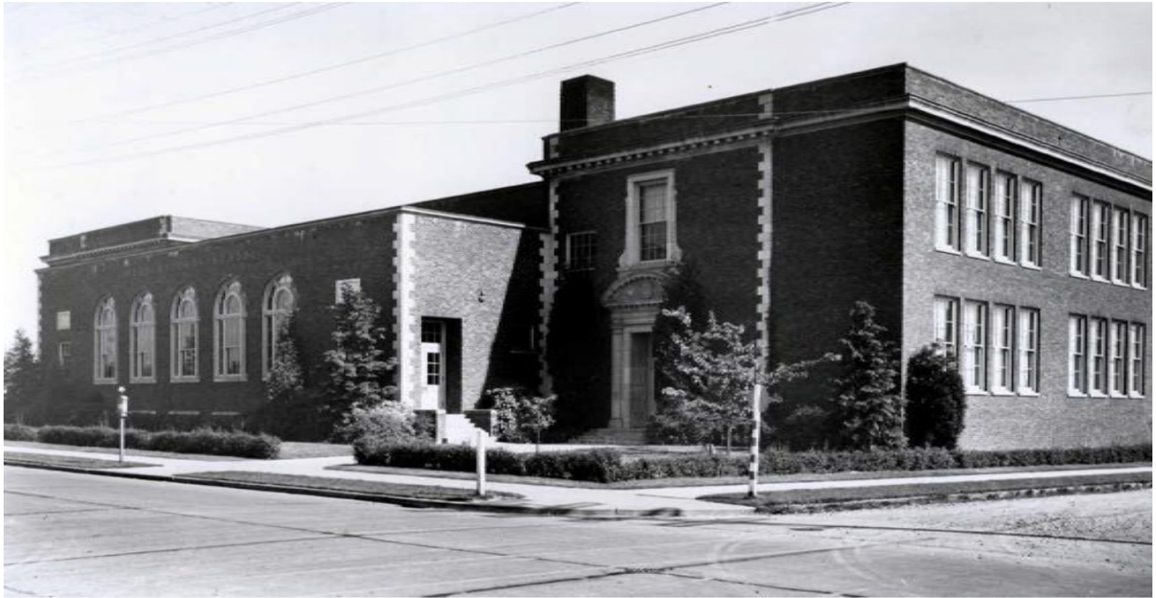
Loyal Heights Elementary School, 2501 NW 80 th Street, 1939
