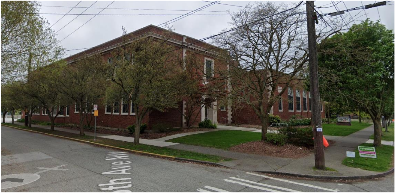
Loyal Heights Elementary School, 2501 NW 80 th Street, 2021
