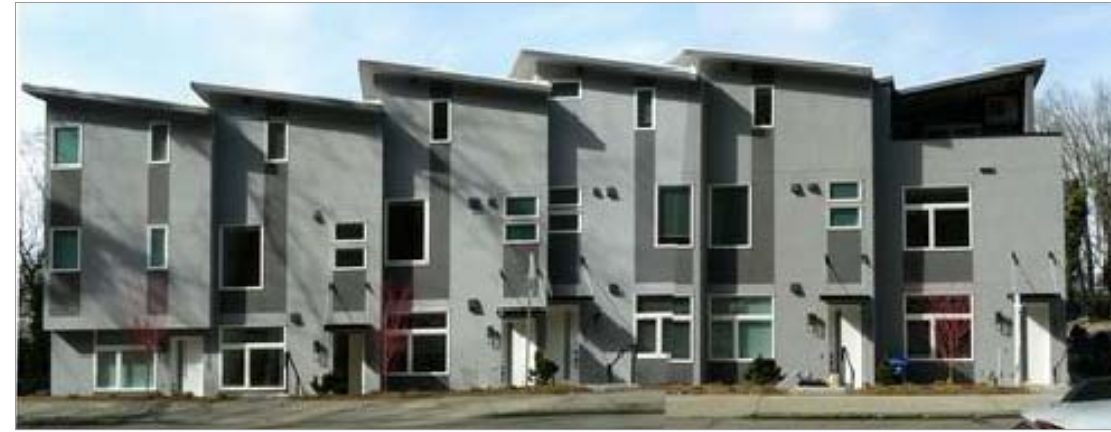
Building West Side of Lakeview Blvd E.
