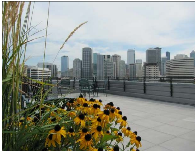
Example of Roof Top Deck
