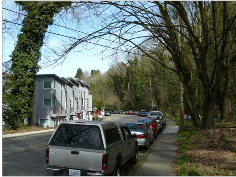
Building West Side of Lakeview Blvd E.
