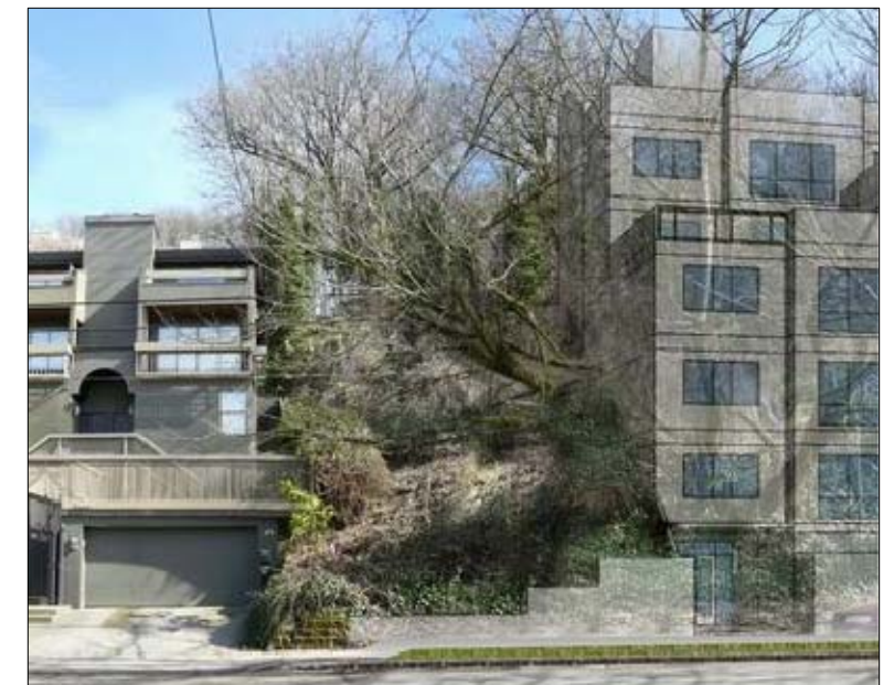
Existing Building Adjacent to Proposed Site
