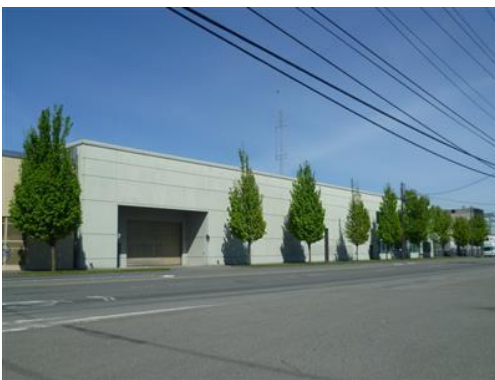
(Source: King County Assessor)
