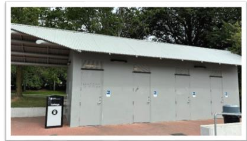
Newly renovated single-stall restrooms at Gas Works Park in 2024
