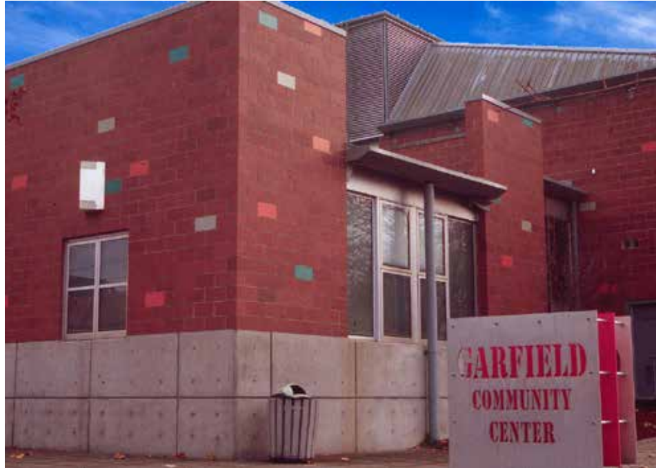
Garfield Community Center
