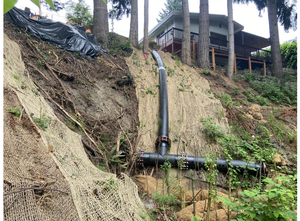
2023 – Temporary culvert installed
