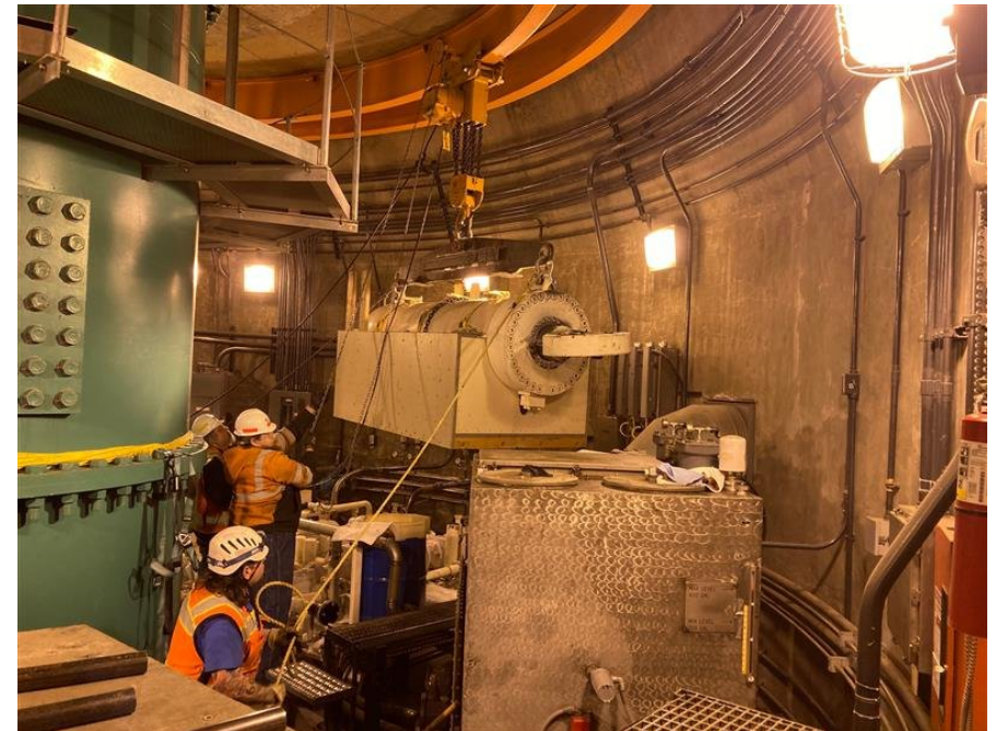
The cylinder is lowered into a custom-built cradle, and removed from pier house using internal crane rails
