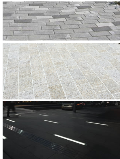
Special Stone Paving with inground lighting
