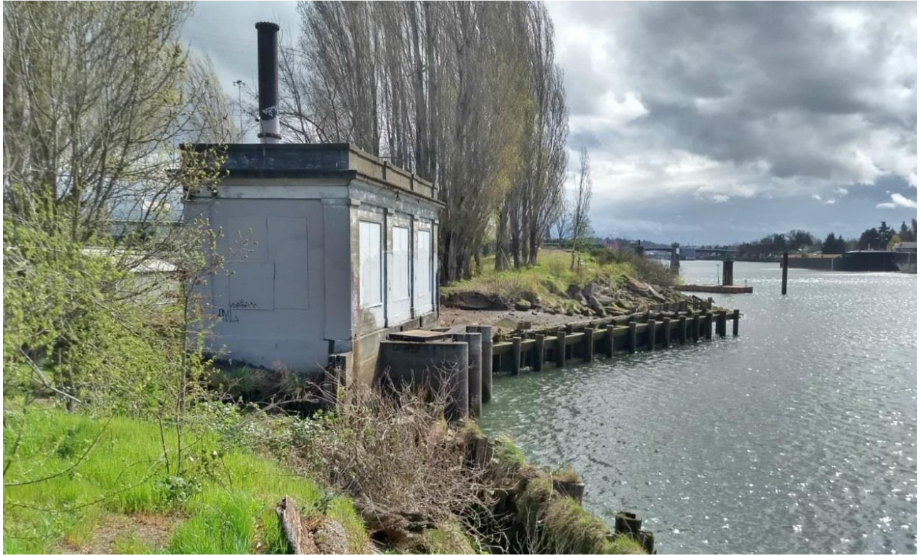
Georgetown Steam Plant Pump House, 7551 8 th Avenue S, 2019
