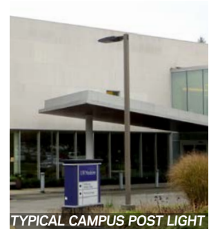
TYPICAL CAMPUS POST LIGHT
