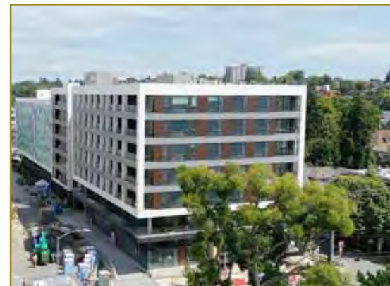
Park Apartments TOD | Seattle, WA
