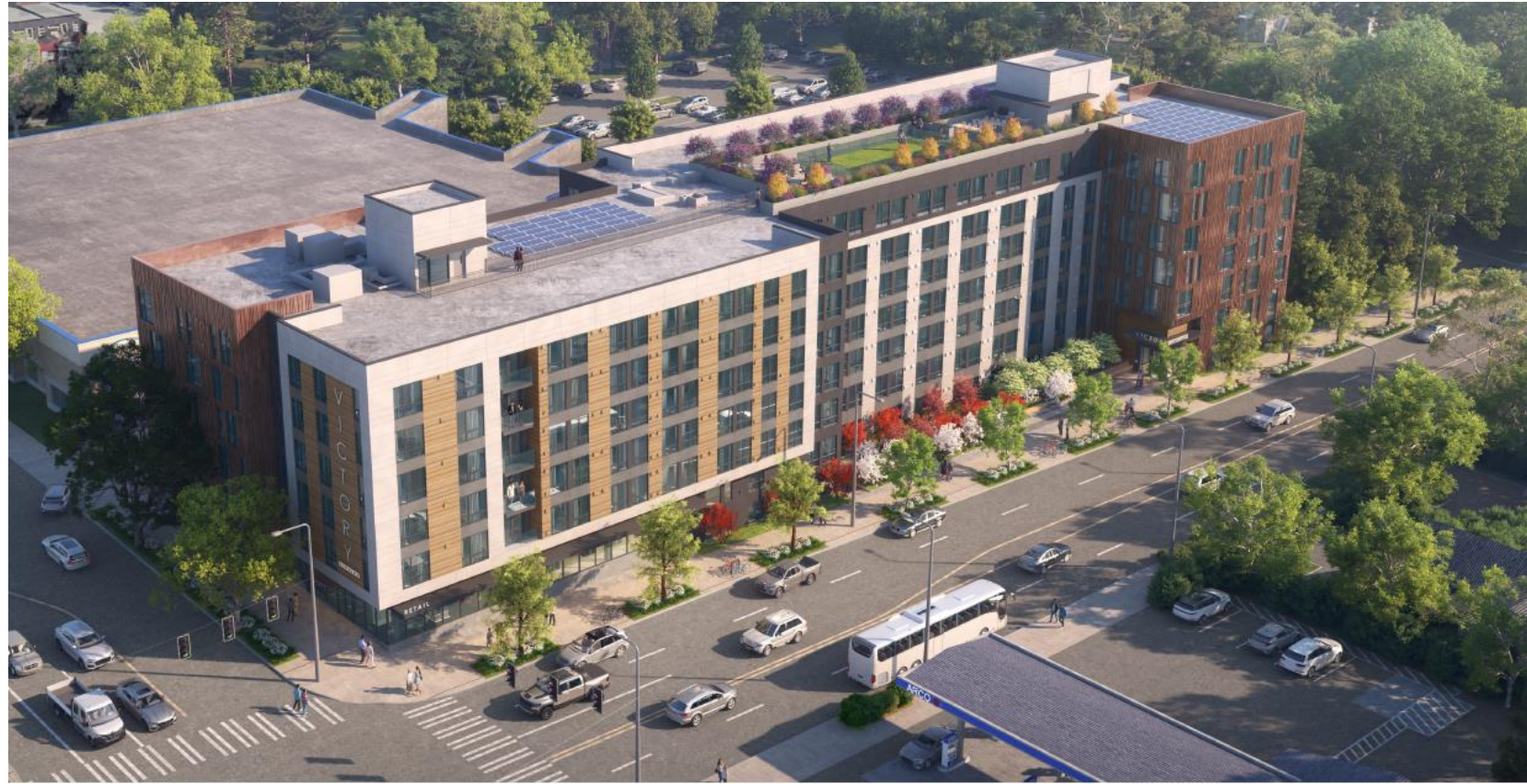
AERIAL VIEW FROM SOUTHWEST
