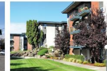
8 PARK AT NORTHGATE APARTMENTS
