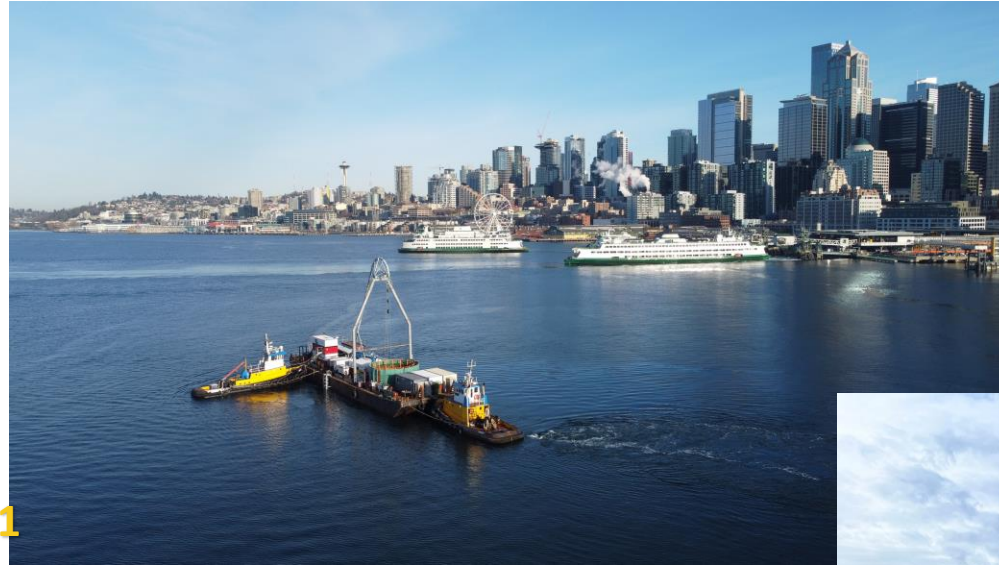
1. Jan 15, 2024: Submarine Cable lay
