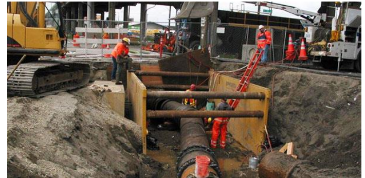
Installing seismic-resistant pipe on S Spokane St
