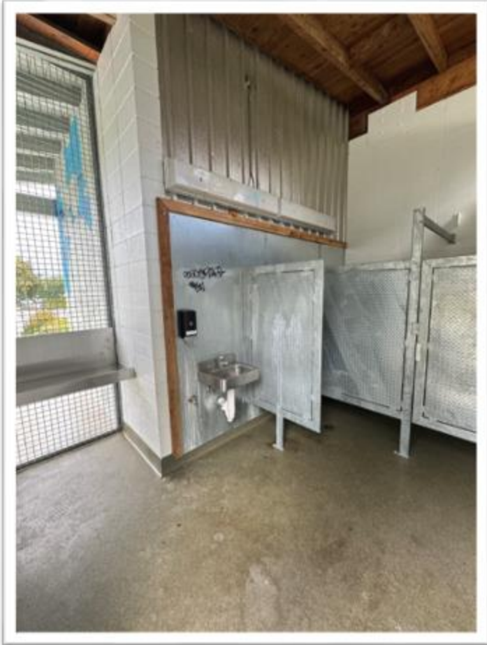
Lakeridge Playground Restroom Weatherization
