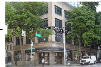
Great Northern Building 1404 4th Ave, Seattle
