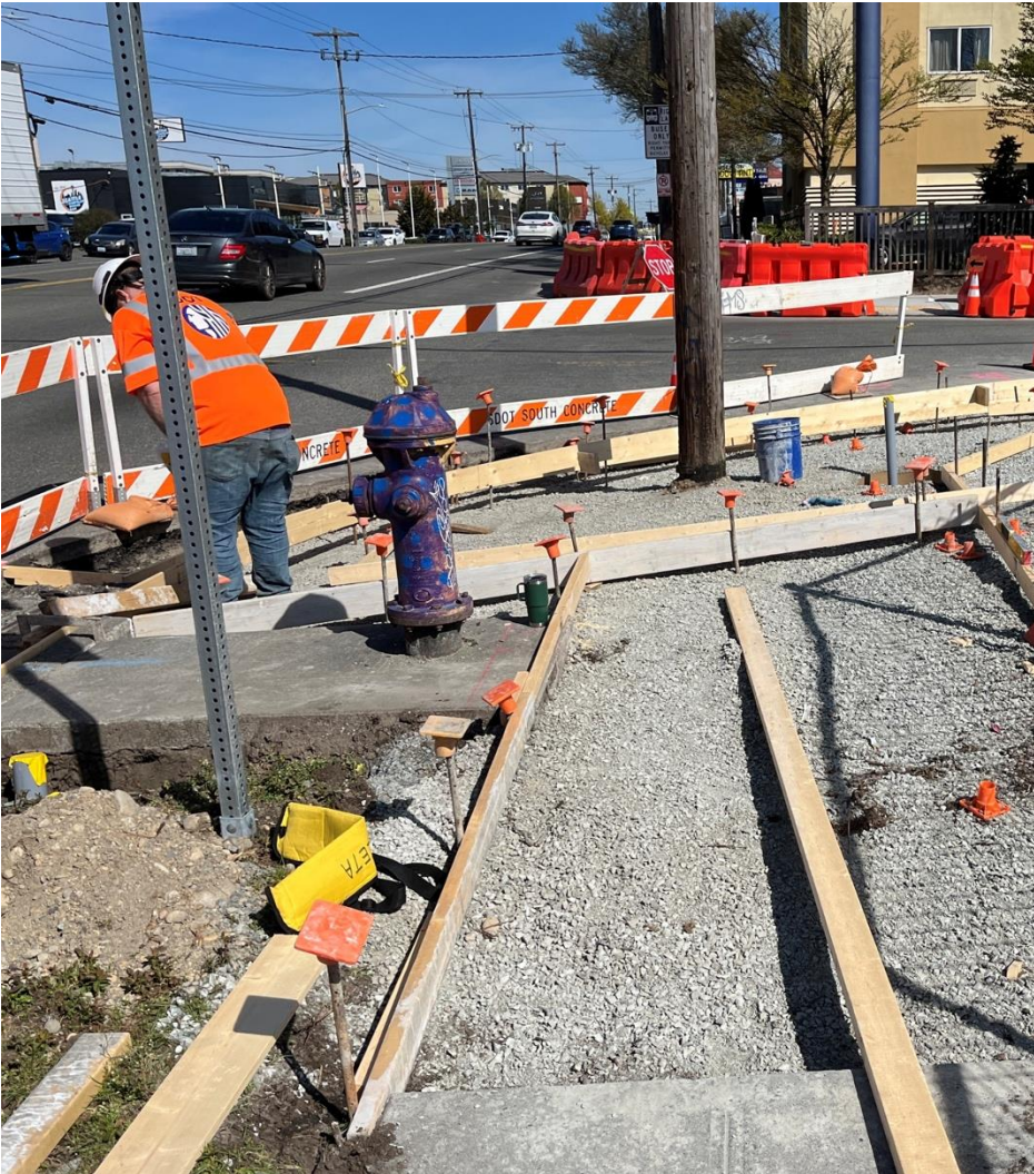
Construction underway at Aurora Ave N & N 137 th St in D5
