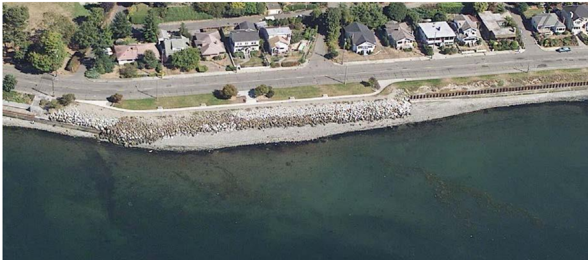
Figure 5. Extent of 1998 seawall failure.
