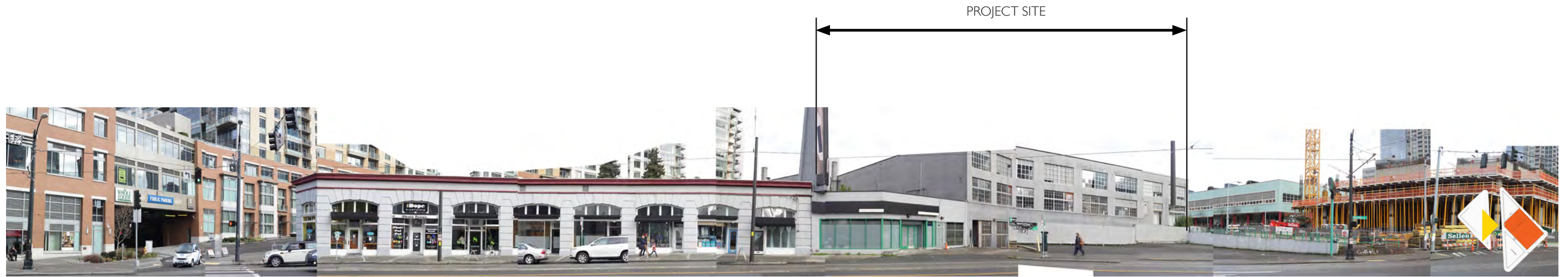
VIEW OF SITE FROM WEST SIDE OF WESTLAKE AVENUE
