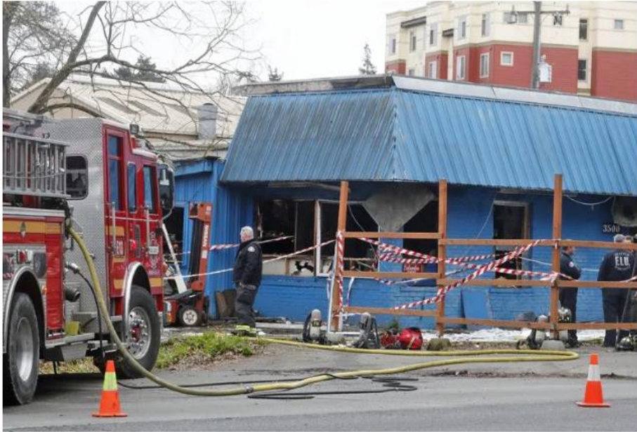
A person was found dead inside this vacant commercial building on Rainier Avenue South where fire broke out Thursday morning. (Greg Gilbert / The Seattle Times) Less ^
