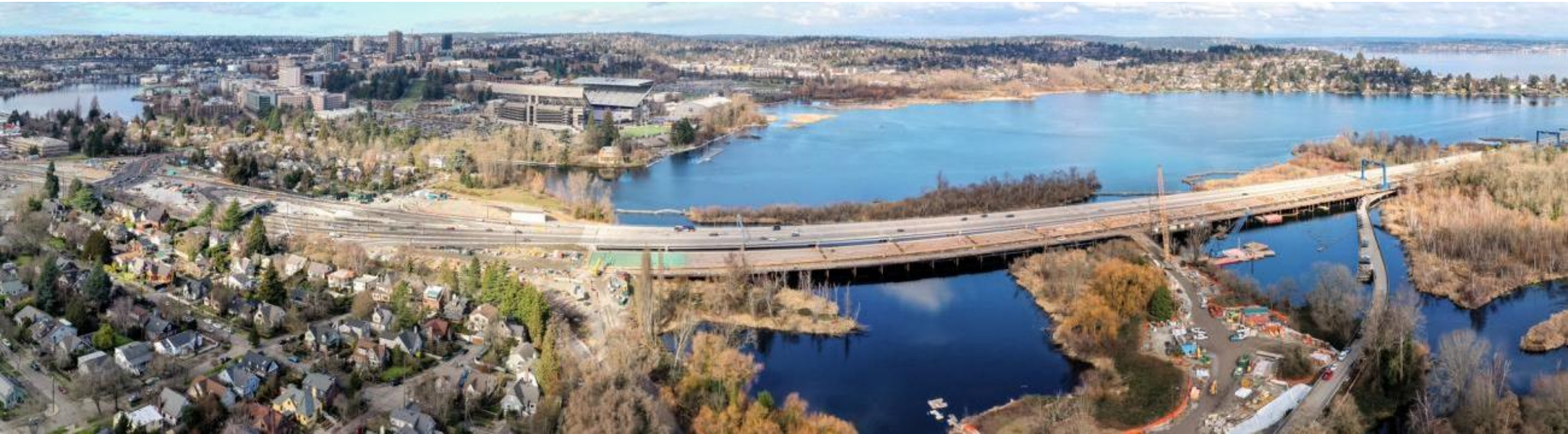
SR 520 Bridge Replacement and HOV Program
