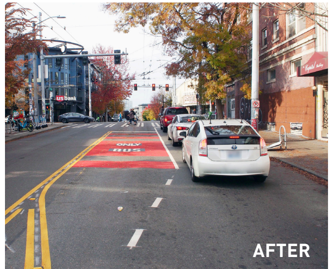
Figure 10. No Turn on Red restrictions, protected left turns, and new pavement markings with bus only lanes was added to the intersection of Broadway & E Olive Way—an identified high collision location—to reduce conflicts between turning movements and people walking and rolling.
