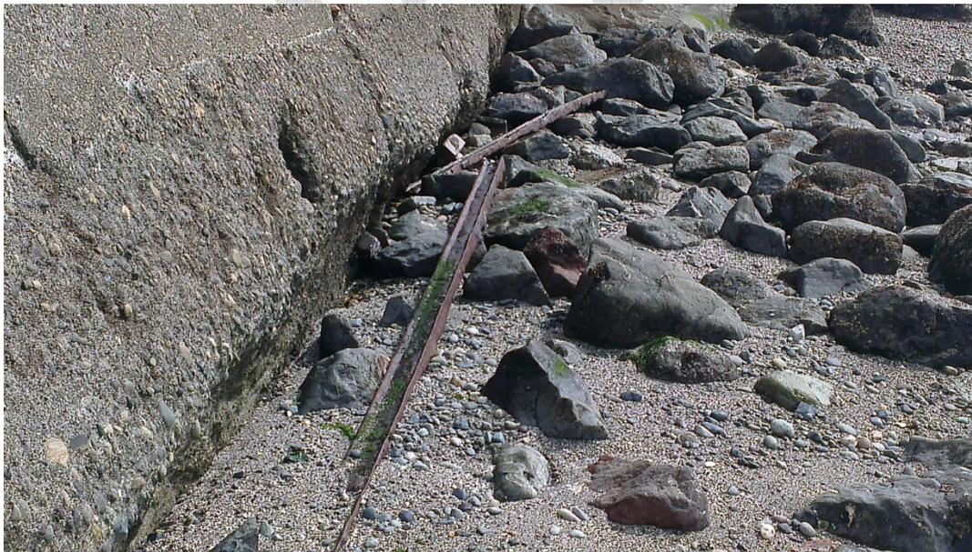
Figure 3. Corroded steel rails and failed top waler which historically held tie back anchors. Also note scour of sediments adjacent to concrete footing.
