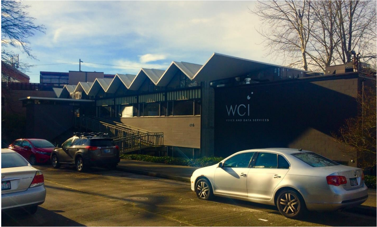
Pacific Architect & Builder Building, 1945 Yale Place East, 2017
