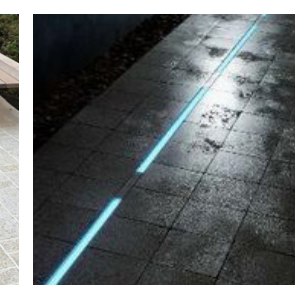
Special Stone Paving with inground lighting
