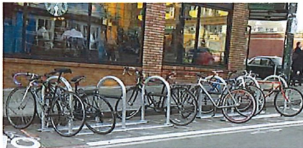
A bike corral with “inverted U” style racks provide ample and convenient parking without impeding a narrow sidewalk.
