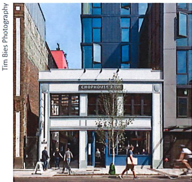
New development incorporates a historic facade and mid-block passageway. The two-story facade provides a transition from the taller building to a pedestrian scale and breaks up the building massing.
