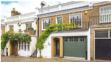
A pedestrian-friendly shared space is lined with balconies, entries, landscaping, windows. The presence of garage doors is minimized.
