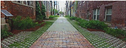
Permeable pavers delineate space along the alley. Landscaping provides a buffer from residential uses.
