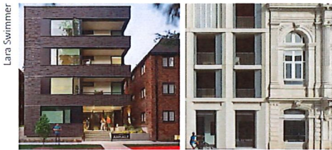
Two examples of new development reflecting context through the use of related materials, datum lines, and horizontal and vertical elements.
