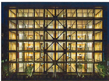
A cohesive design expresses the modular construction technology used for this project.
