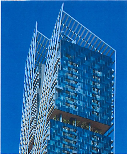
A sculptural roof line reinforces the design concept and transitions to the sky.
