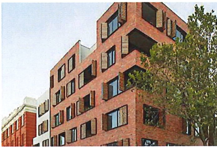
Operable windows at upper-levels add human scale with an ever-changing facade. The notched parapet and corners breakdown bulk of the form.
