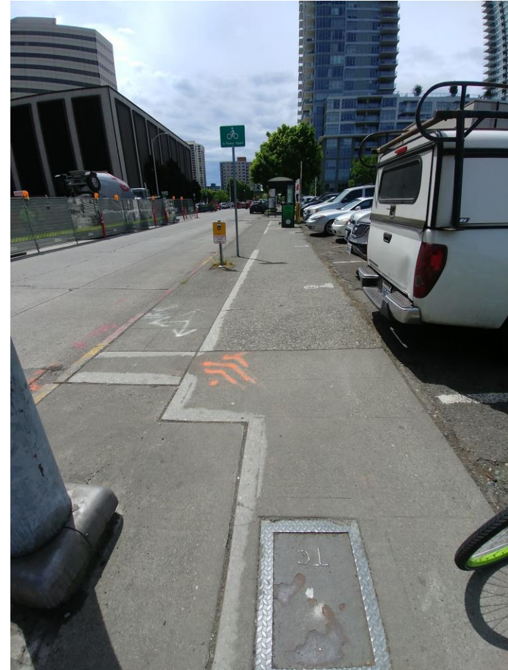
Example of a beveled sidewalk in Belltown
