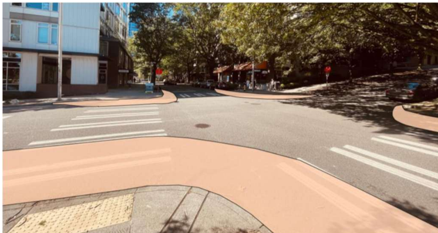
3) Pedestrian improvements at 8 th Ave & Marion St.
