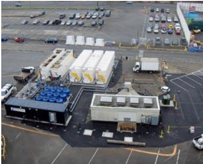
South Park Water Quality Facility
